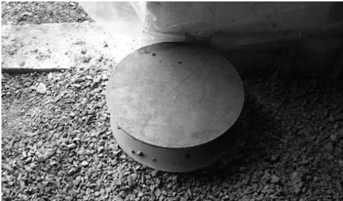
PNA bollard base on level subgrade
