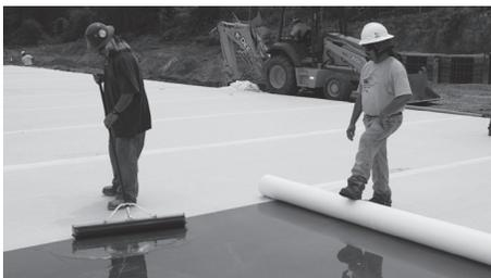
Easy to roll out and lay flat on the slab
