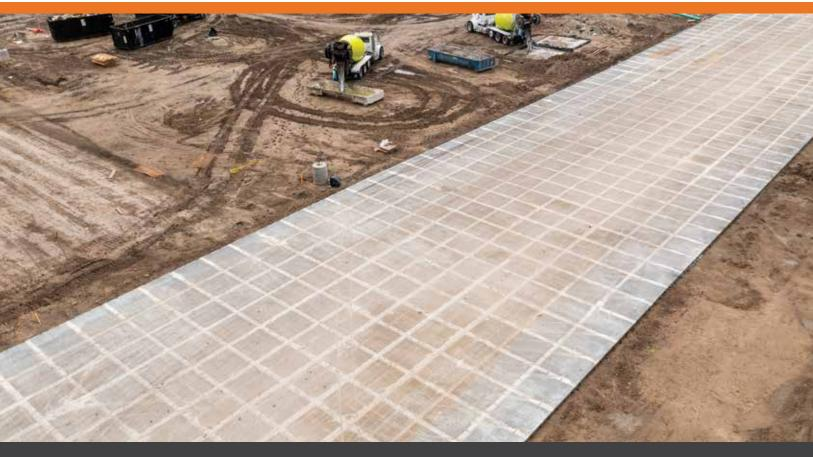
With a joint layout optimized by our OptiPave2 software, curling is reduced and axle loads are better distributed, reducing out-of-joint cracking.
