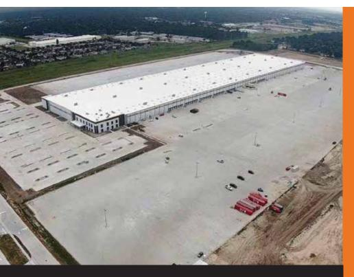
The largest TCP project at it's time of completion, a high performance TCP design reduces the amount of concrete needed.
