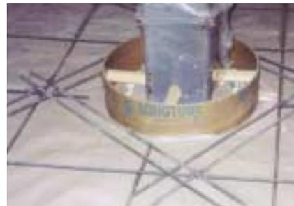
Conventional dowels have to be removed to allow for the removal of edge forms. They then must be replaced before the adjacent slab is placed. Unless workers take extreme care
