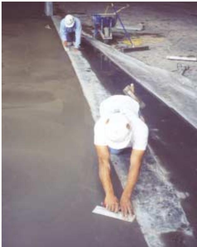
**Above: Additional reinforcement in column detailing provides protection against re-entrant cracking. Left: Hand troweling of the joints ensures that the joints are flat.**
