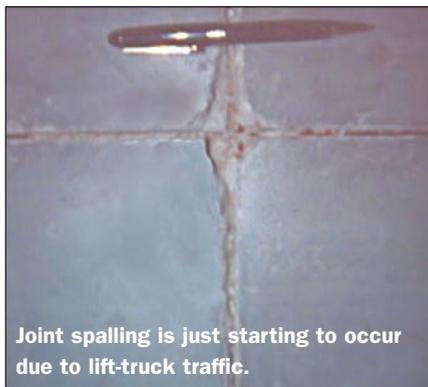
Joint spalling is just starting to occur due to lift-truck traffic.
