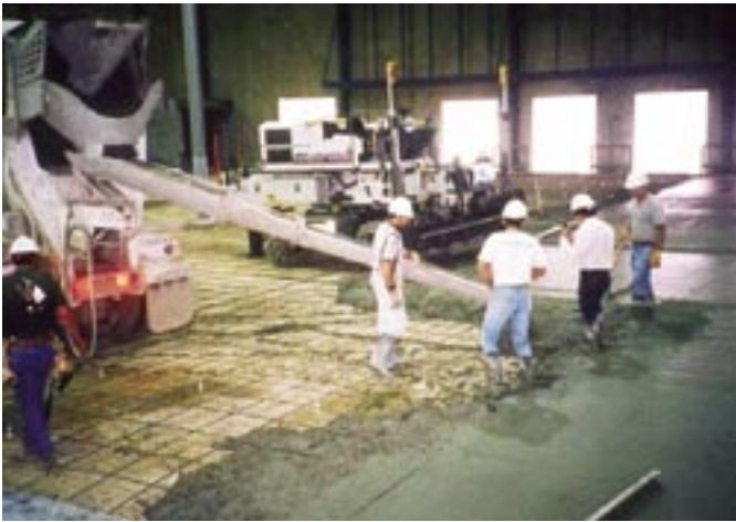
Fig. 1: Light reinforcement continued through contraction joints for load transfer and chaired up just prior to concrete placement and screeding
