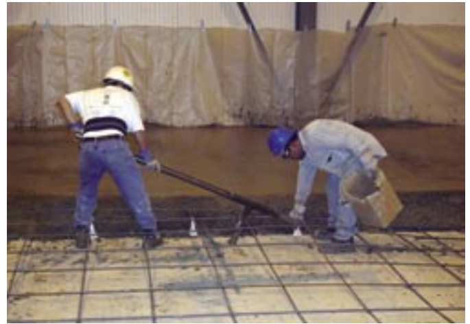
Fig. 1: Light reinforcement continued through contraction joints for load transfer and chaired up just prior to concrete placement and screeding
