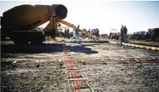
Fig. 2: Plate dowel baskets for contraction joints are installed over painted lines and placed in saw-cut joints just prior to concrete placement and screeding
