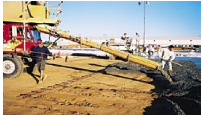
Fig. 2: Plate dowel baskets for contraction joints are installed over painted lines and placed in saw-cut joints just prior to concrete placement and screeding
