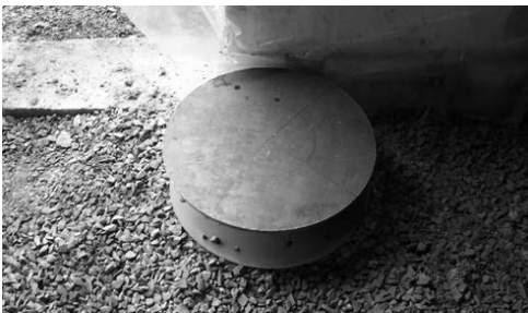
PNA bollard base on level subgrade
