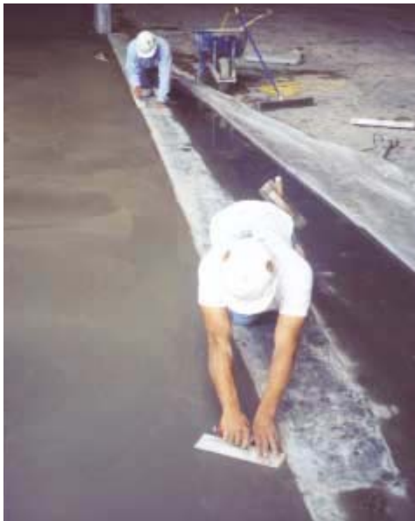
Above: Additional reinfocement in column detailing provides protection against re-entrant cracking. Left: Hand troweling of the joints ensures that the joints are flat.
