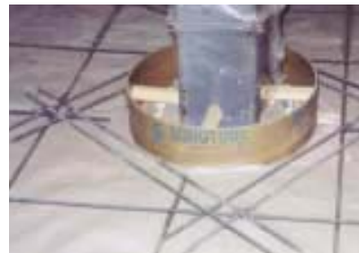
Above: Additional reinfocement in column detailing provides protection against re-entrant cracking. Left: Hand troweling of the joints ensures that the joints are flat.
