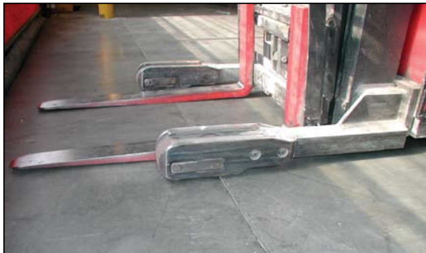
Figure 1: The use of the new style lift trucks with small, hard wheels requires better slab designs to prevent joint spalling
